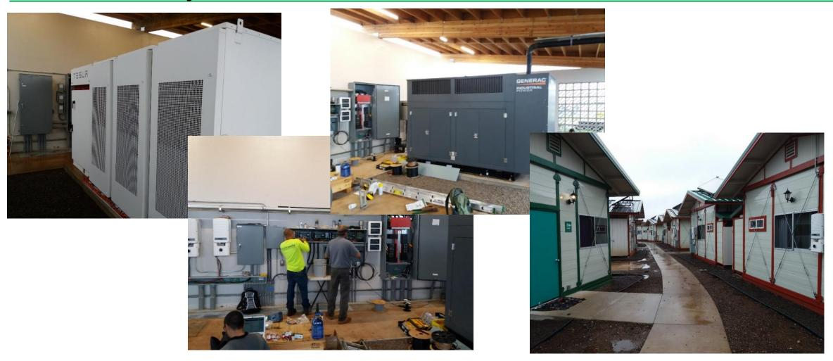
ASC-4 Battery. Hawaii, Feb 2018. 200 kW PV capacity, a 150kW genset capacity, a 150kW/610kWh electrical storage and a 25kW utility incoming.
