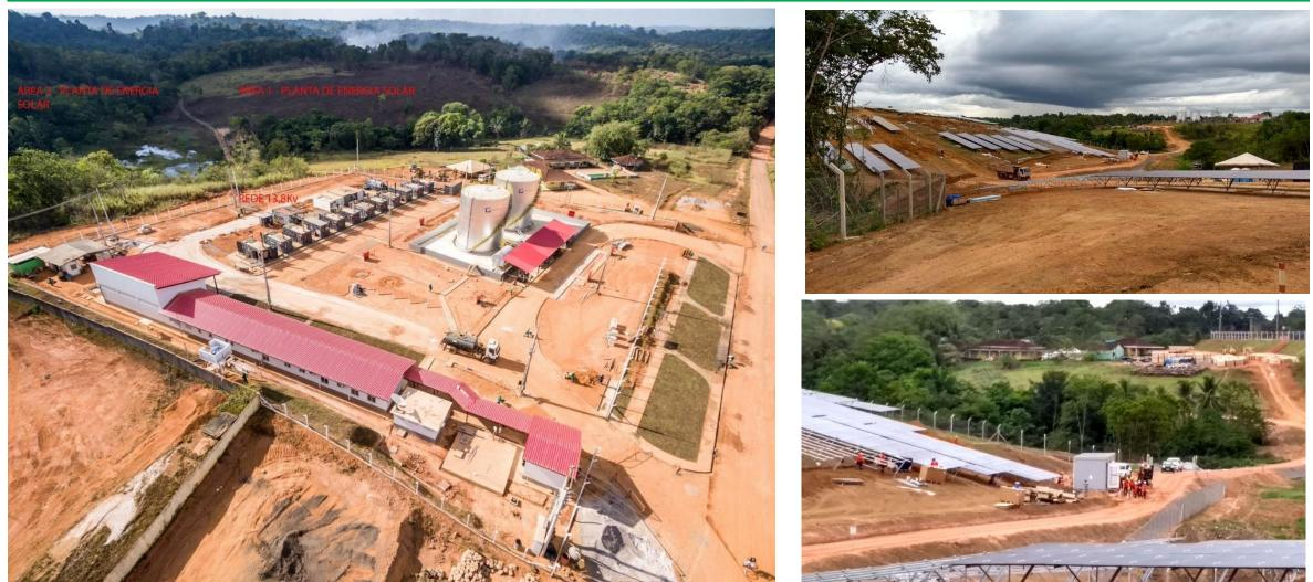
ASC-4 Solar. Brazil, Dec 2017. 4 MW PV capacity, 12 MW genset capacity and a Reuniwatt forecast system. It's purpose is to reduce the use of diesel and supply power to Oiapoque city and rural areas.
